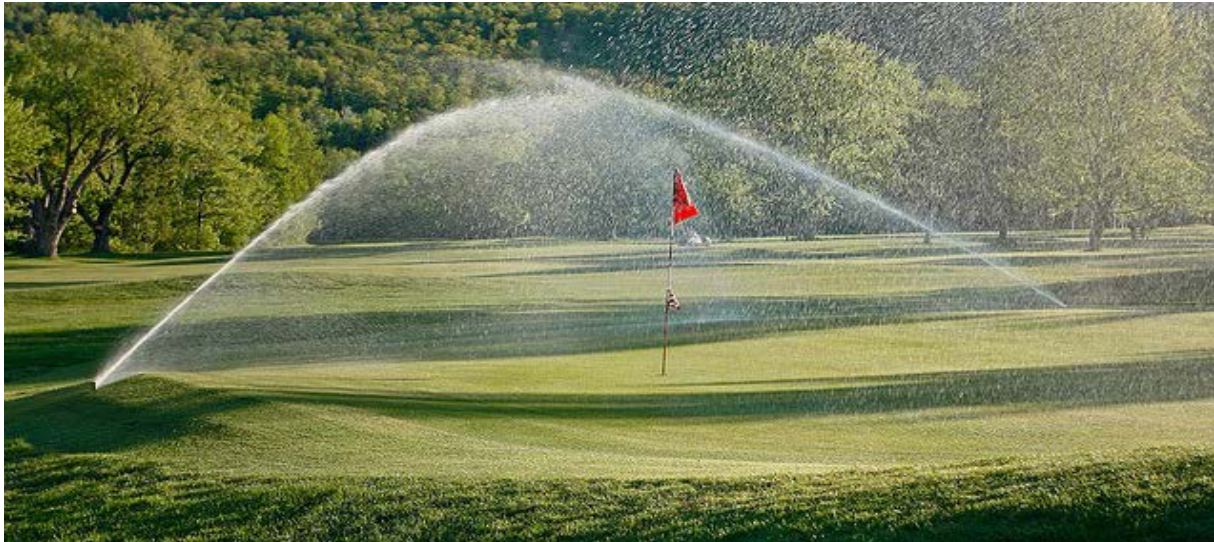
Fig. 20 Sprinkler irrigation for turfgrass (rotor pop-up sprinklers in a golf field)
