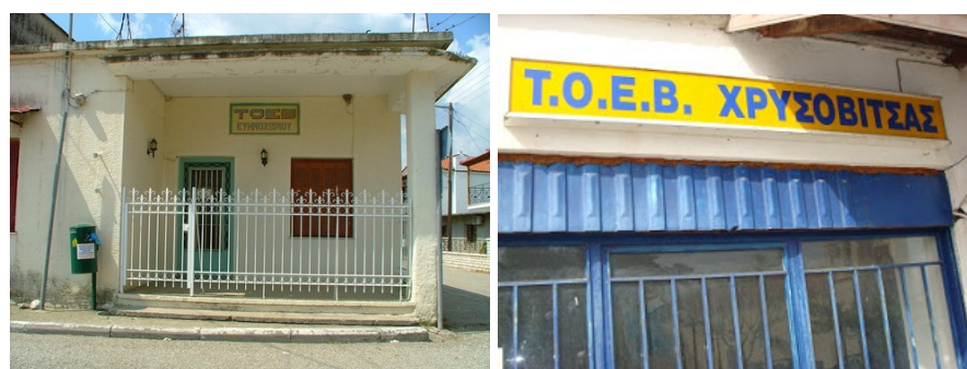
Fig. 13 Typical offices of Local Organisations of Land Reclamation in the area
