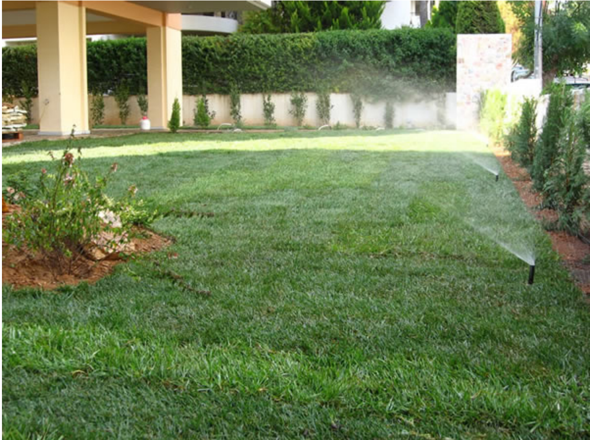
Fig. 66 Sprinkler irrigation for turfgrass (spray pop-up sprinklers)
