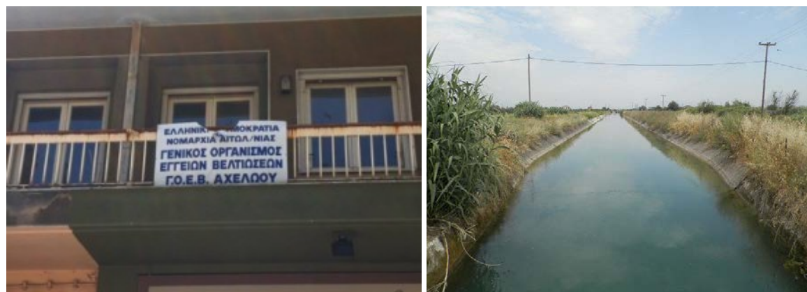
Fig. 11 The offices and an indicative canal of the GOLR of Acheloos at Agrinio
