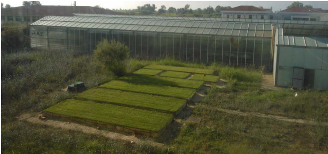
Fig. 15 Construction of the experimental setup and a general view from NW
