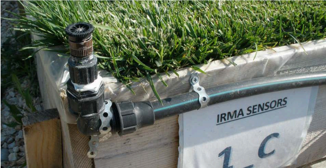
Fig. 19 Sprinkler placement in each 2x6m container
