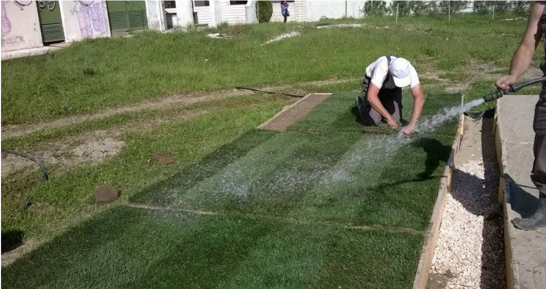
Fig. 18 Installation of sod
