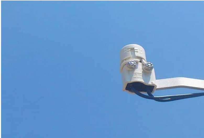
Fig. 23 Hunter Mini-Click, rain sensor
