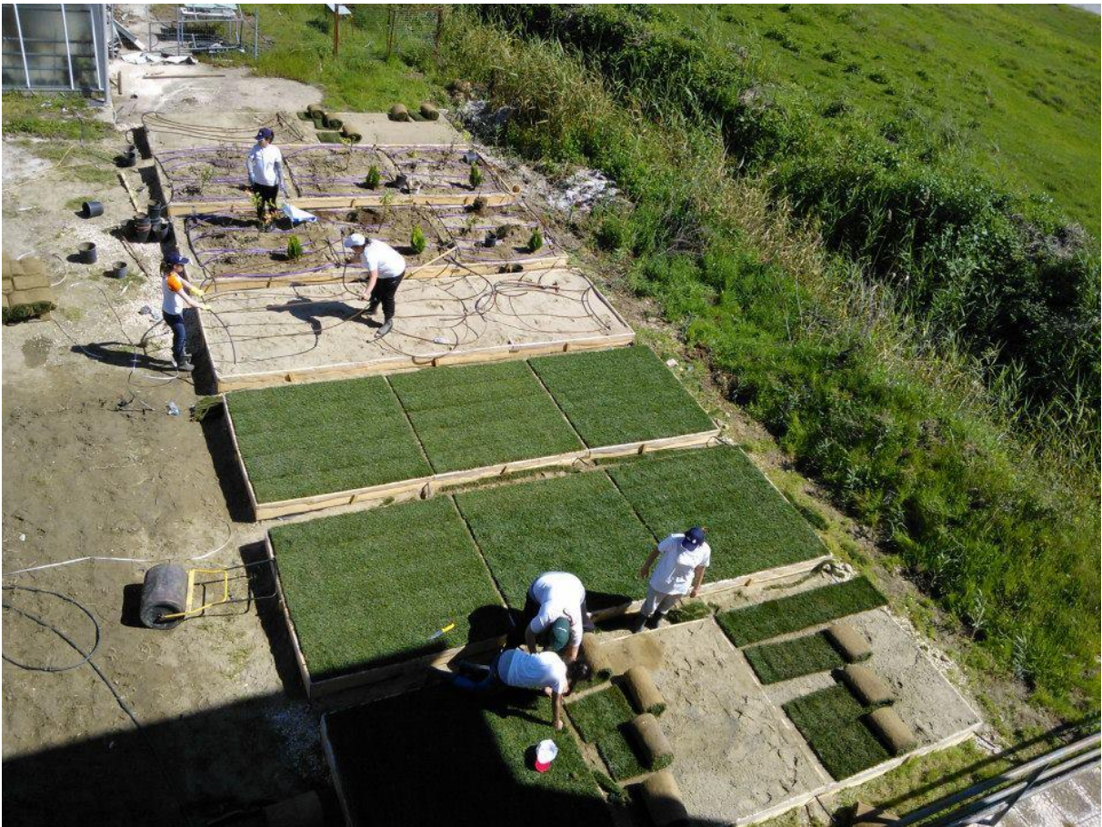
Figure 7 Indicative stages from the construction of the experimental setup
