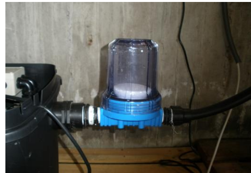
Figure 12 Chlorinating device
