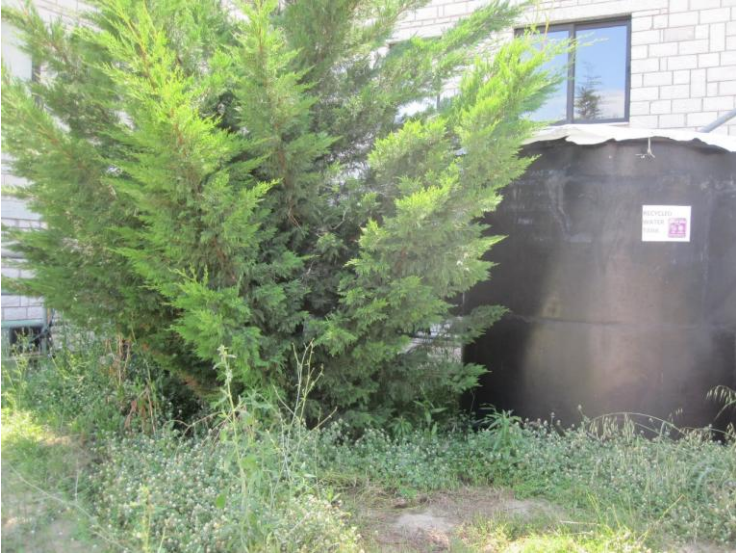
Figure 15 Site of storage of recycled water
