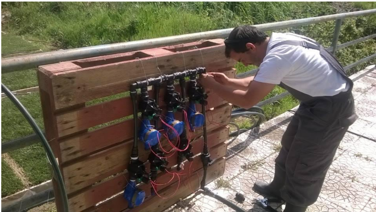
Figure 8 Construction of the irrigation system head (initial placement)
