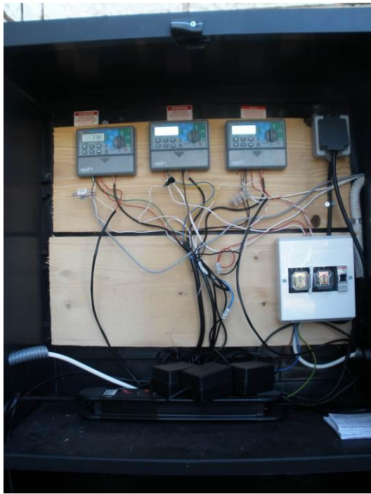
Figure 18 Controllers and rain sensor
