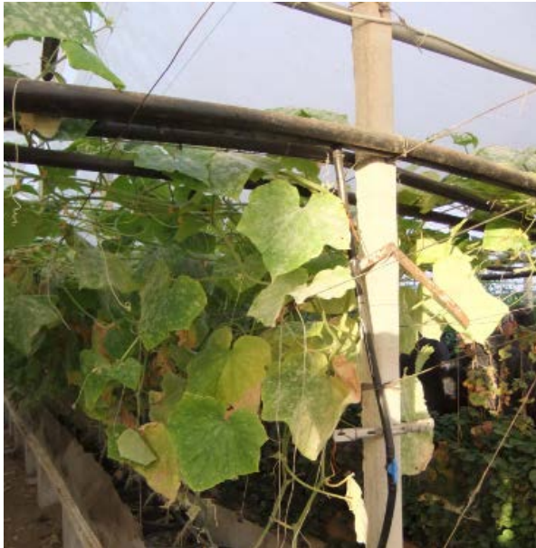
Fig. 58 Irrigation problems in greenhouses (leakages in junctions between secondary pipes and tertiary)
