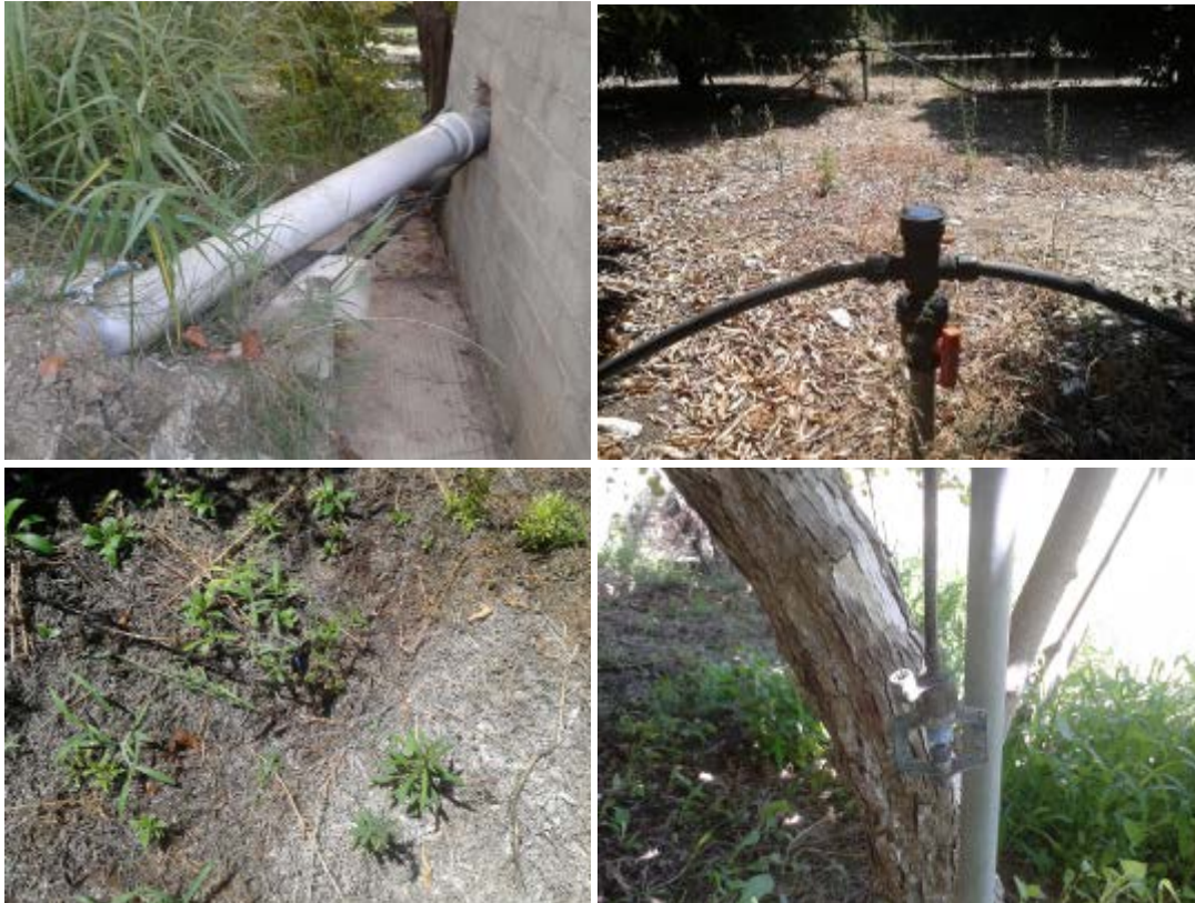
Fig. 34 Irrigation pipes main pipes, secondary and tertiary
