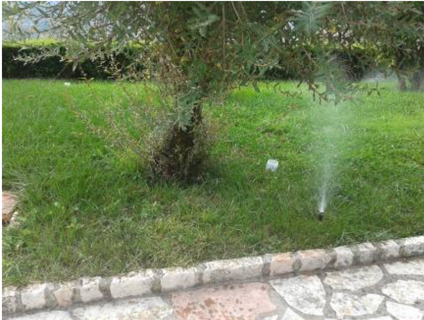
Fig. 71 Wrong irrigation process
